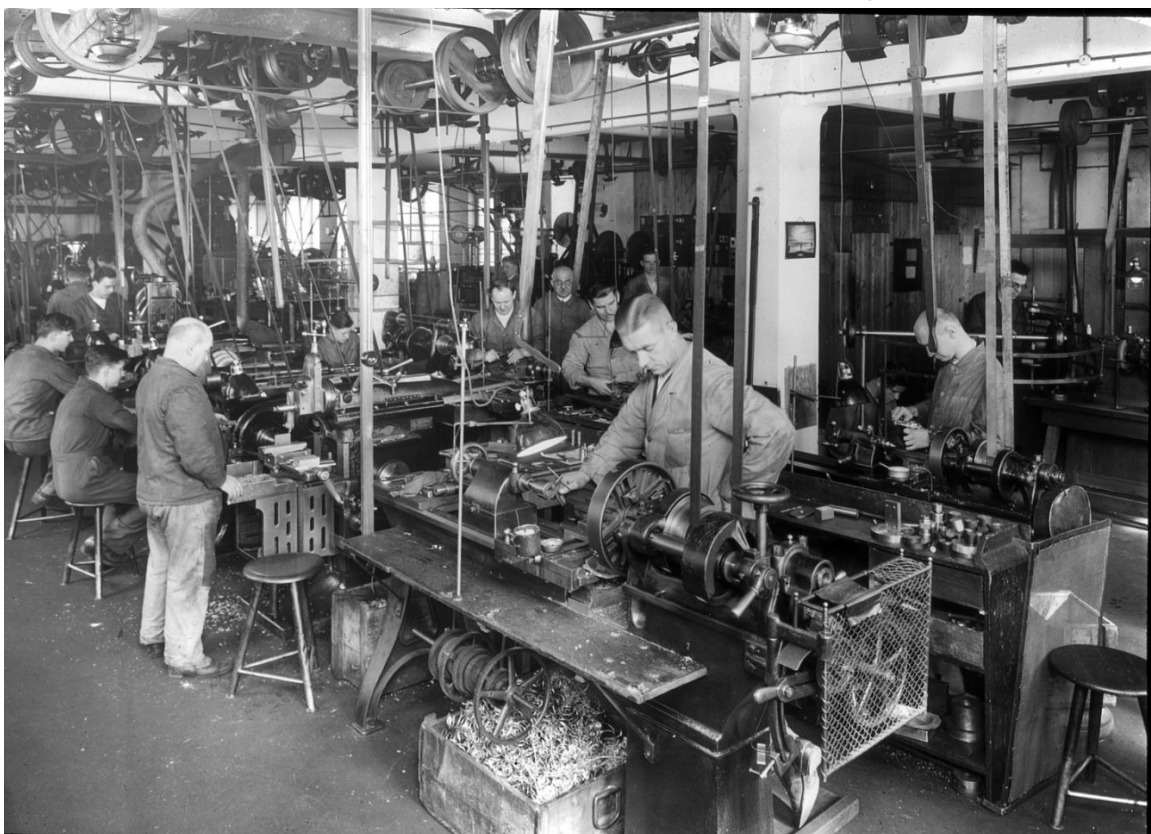
This 1934 photograph shows the system of overhead shafts driving machinery by belts at 24 Schandauer Straße
